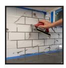
Grouting can begin immediately. **Use only un-sanded or non-sanded grout.** Apply grout in the exact same manner as you would when working with ceramic tile using a rubber float. Use a clean damp sponge to remove excess grout, then use a damp micro fiber towel to wipe off grout residue. If desired, grout matching caulk can be applied in the corners and where the tile board meets another surface, such as the countertop.
