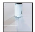
Cutting the tile: Access holes for pipes and fixtures
