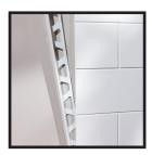
**Step 4:** Edging can be installed by first measuring the length needed for each edge, then install by sliding the edge trim under the installed tile before the glue sets. This same process is performed if edging is also applied along top of the tub enclosure. Refer to the edging manufacturer's instructions regarding inside and outside mitered corners.
