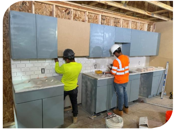
Figure 4: Installation of ceramic backsplash with 2-person crew
