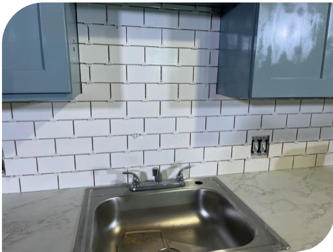
Figure 6: Spacers in-between ceramic tiles during setting period
