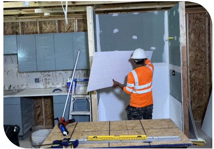
Figure 7: 1-person crew installation of Six3Tile shower kit
